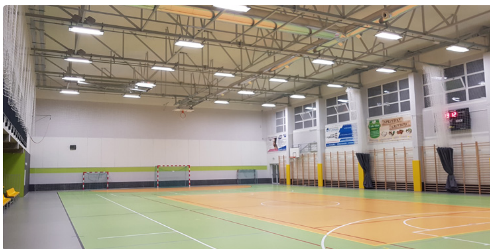
Photograph 2.34. The Entertainment and Sports Hall in Ryczywół
