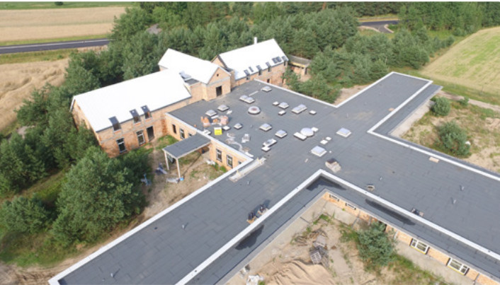
Photograph 2.17. The in-patient hospice building under construction in Michałowo municipality
