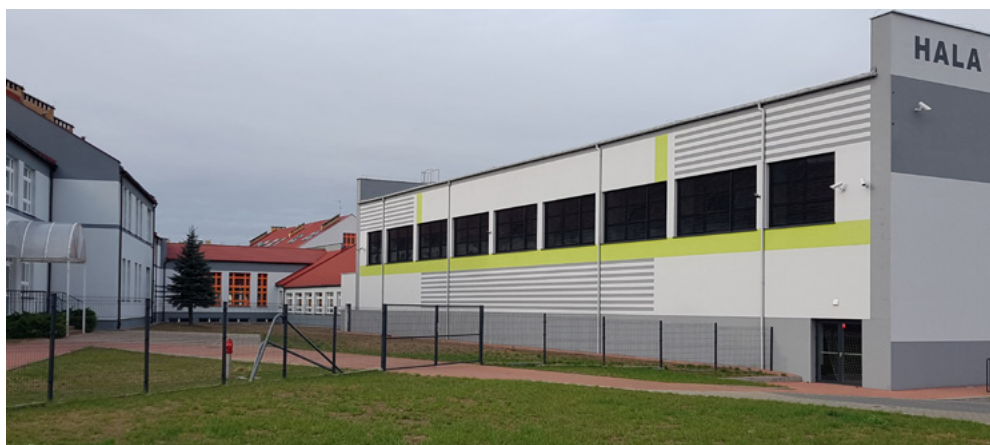
Photograph 2.33. The Entertainment and Sports Hall in Ryczywół
