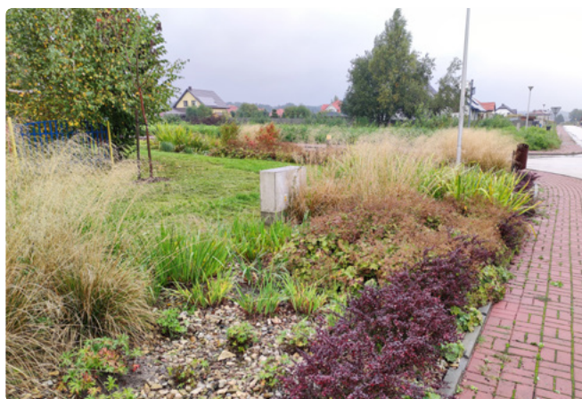
Photograph 2.20. The rain garden in the area at risk of flooding in the centre of Piaseczna Górka
