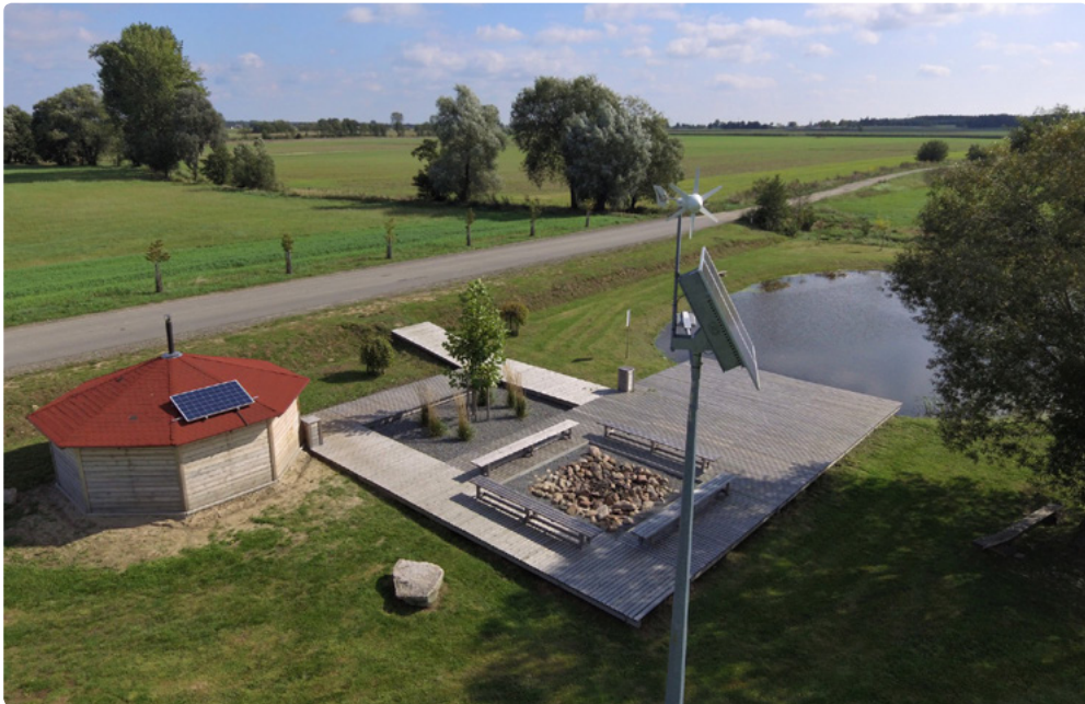
Photograph 2.5. A view of the pond and shed in Łuszczanów
